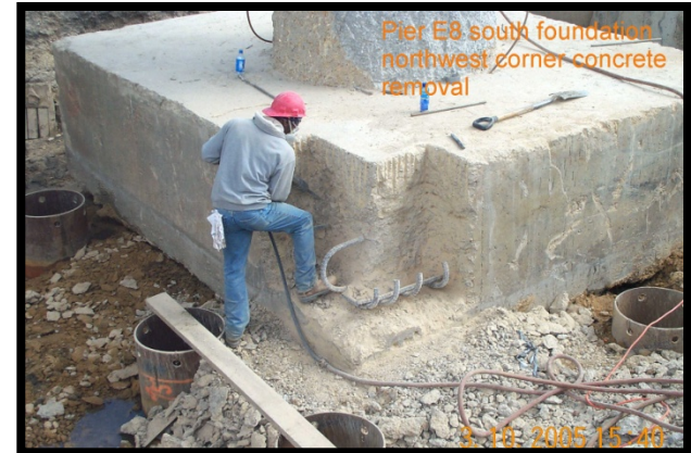
Foundation Demolition
